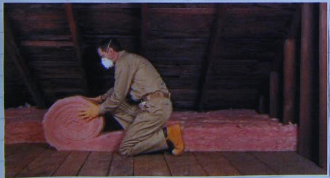
Installation of the fibre glass wool loft insulation.
